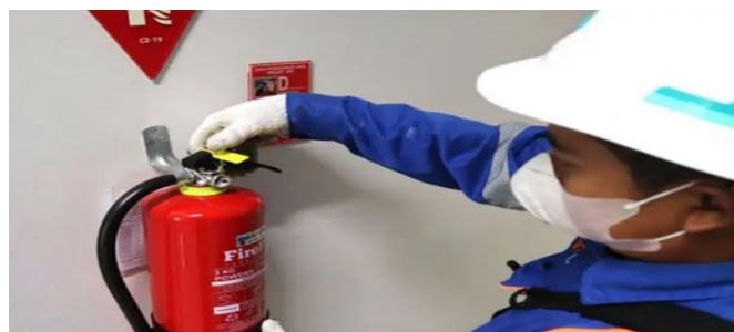
Figure 16. Replacing the APAR
